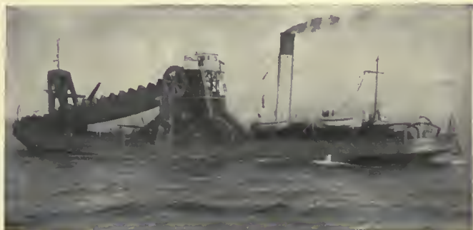
FIG. 10.—Hopper-dredger, "David Dale," with buckets of 54 cub. ft. capacity (see fig. 11) built for the North Eastern Railway Company by Lobnitz & Co.
